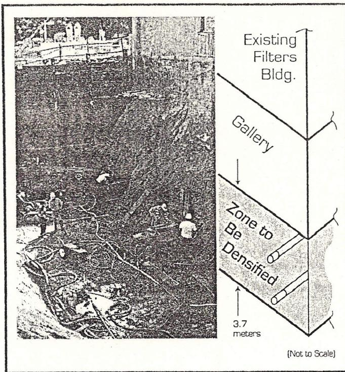
Fig. 3: On-Site Details During Compaction Grout Operation and Section through the area to be compacted
