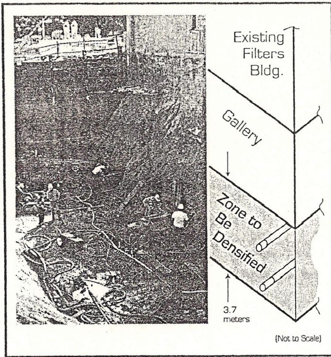
Fig. 3: On-Site Details During Compaction Grout Operation and Section through the area to be compacted
